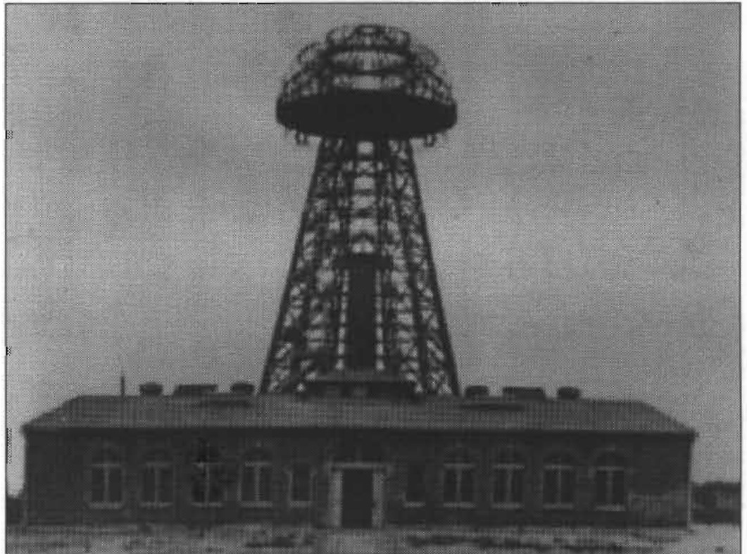
The 167-foot-high transmitter at Wardencllyffe, erected for purposes of "world telegraphy" in 1901.
